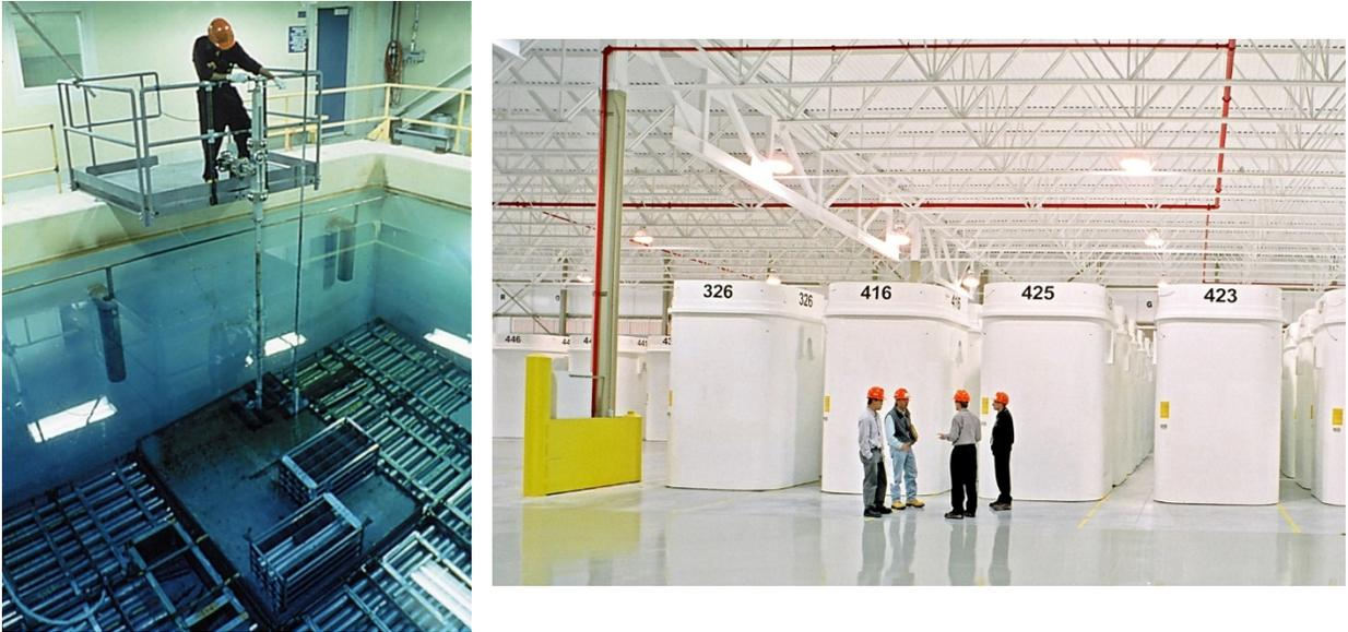
**Figure 2.3: Photos of workers in CANDU used fuel bay and in dry storage facility.**
