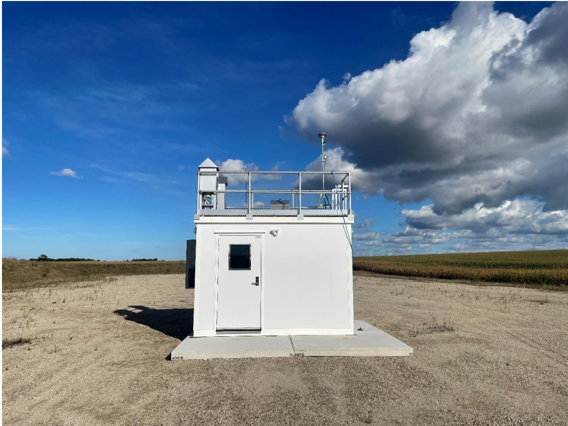
Figure 7-8: Atmospheric Monitoring Station at Borehole 1
