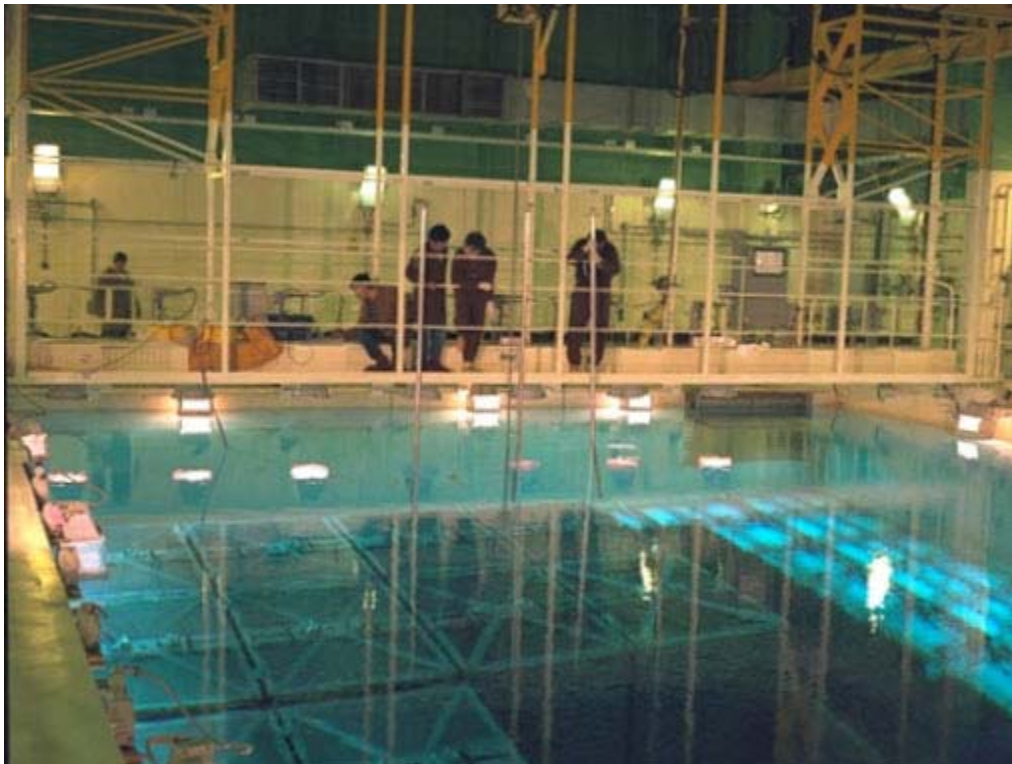
Figure 2-3: Water-Filled Waste Fuel Bay
